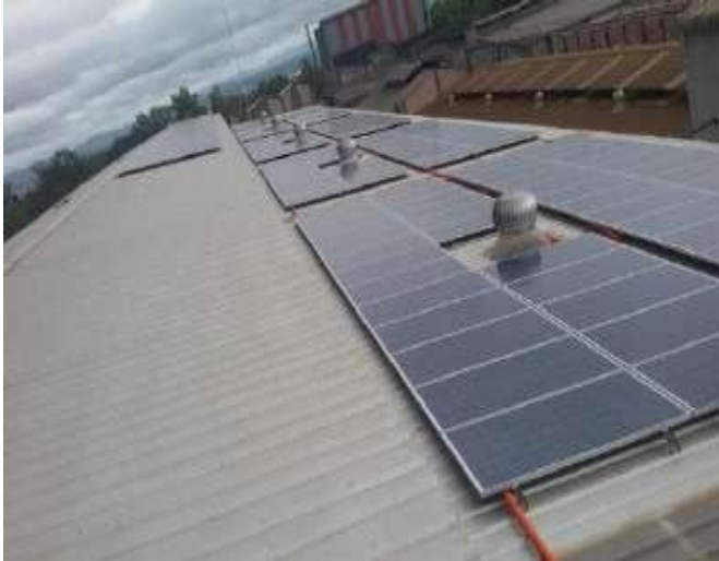
100 KW Roof top static solar cell installed in hall number 7
